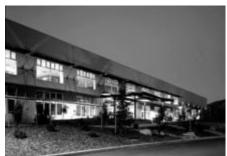
Light shelves (on the lower level) and shading devices help make this conventional tilt-up concrete building energy efficient. - Photo Credit: Miller/Hull
